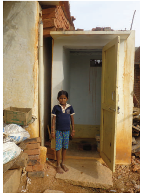
Toilet built by women of ATDDT, Keeranur
